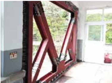
Site Applying Steel Brace Construction Method (Seismic Reinforcement Method)
